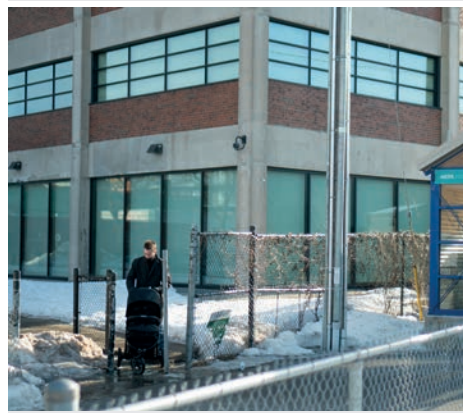
The unfinished crossing at the Parc ARMT station still an obstacle to many Photo: Matias Brunet-Kirk
