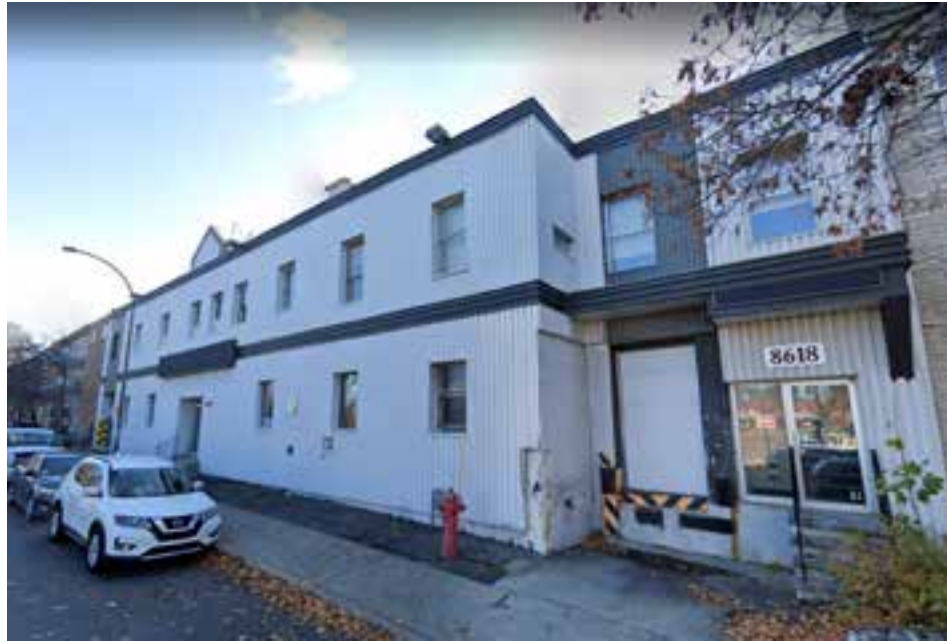
A demolition permit was granted for 8600 de l'Épée to make way for a new social housing project.
